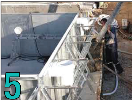
5 Concrete laying to supports
