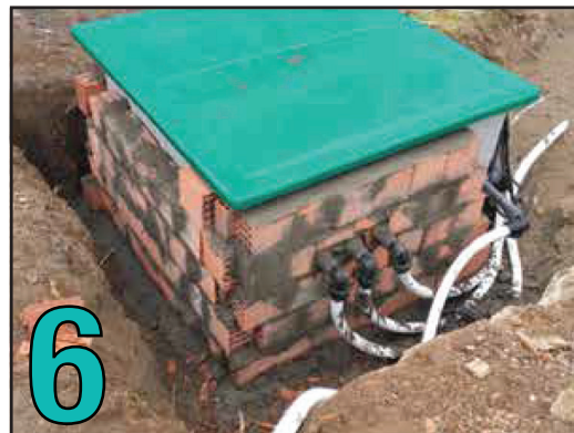
6 Preparation and protection of machine room.
