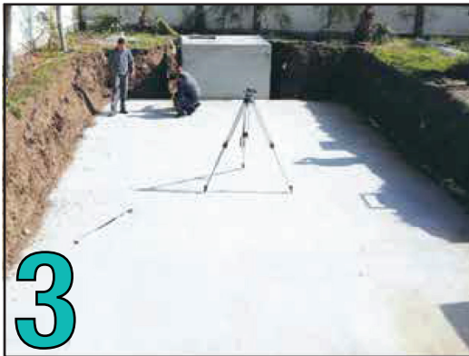
3 Substructural concrete laying
